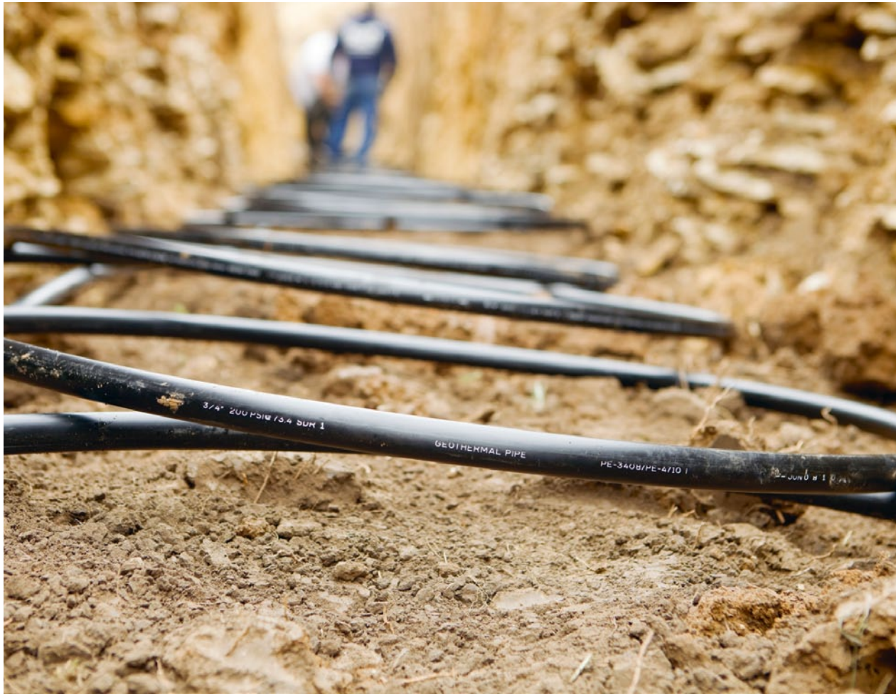
Ground heat collectors take up the thermic energy saved in the underground and transport it to the heat pump
